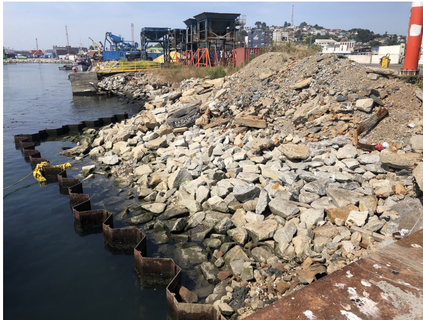
Figure 2.4: Rubble still present between Sitio 1 and 2 after the collapse of the quay during the 2010 earthquake.
