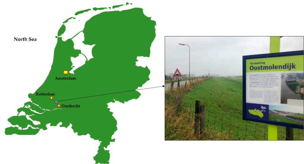
Figure 7. Location of the case study embankment Oostmolendijk.
