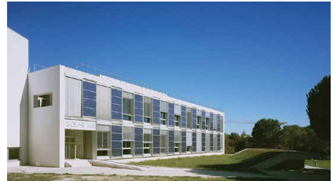
Fig. 8 Solar Building XXI in Lisbon (Portugal).
