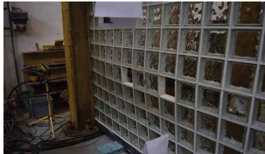
Fig. 12 The wall after the test.
