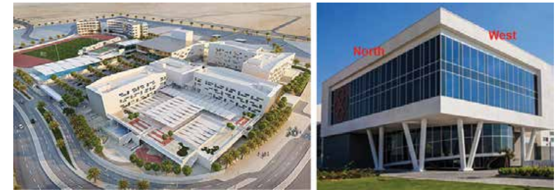
Fig. 1a: SISD Campus general view (Rendering | ARCHILAB – Gabriele M. Rossi Sa), 1b: 110 square meters of electronically tintable glass installed in the façade of the offices at SISD, Architect: ArchiLab, DSA, UA, Source: dubaioursandbox.com
