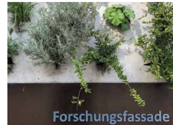
Fig. 9 Detail of the Green Façade at the Frankfurt University of Applied Sciences
