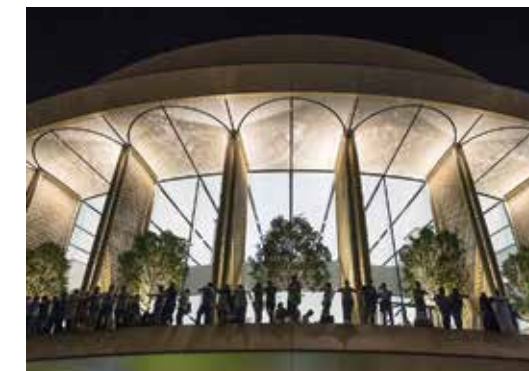
Figure 1: Installed shading system during store opening. Photograph – Nigel Young, Foster + Partners.
