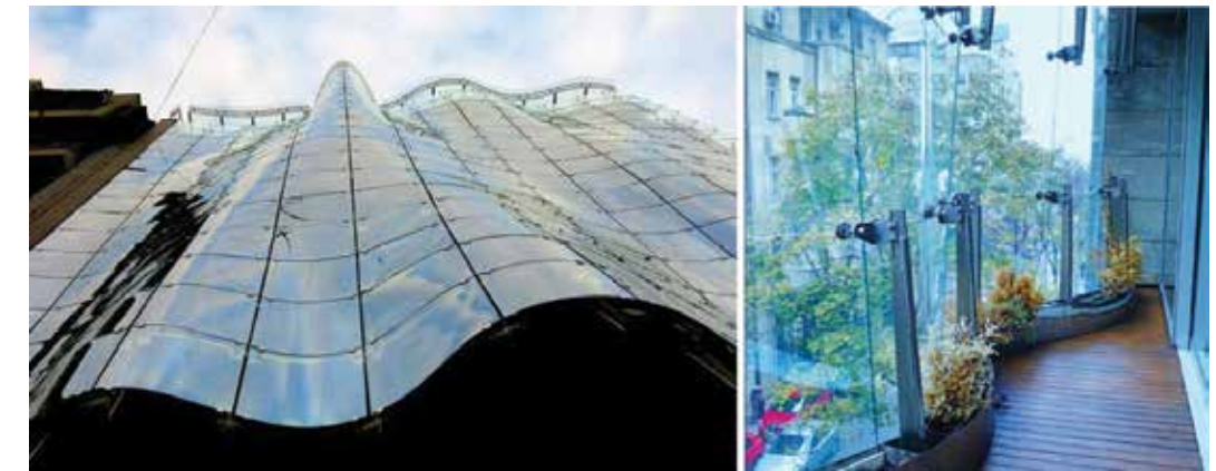
Fig. 1a) and b) Appearance of glass facade of the residential building Infinity.
