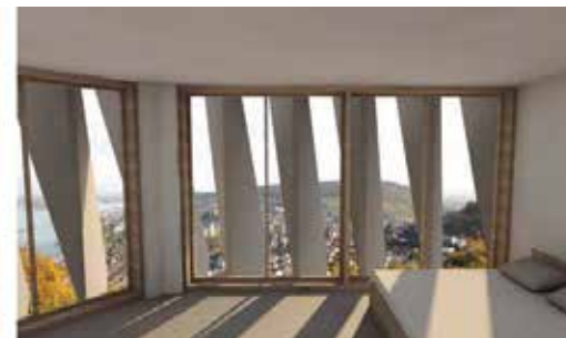
interior view with half closed flaps
