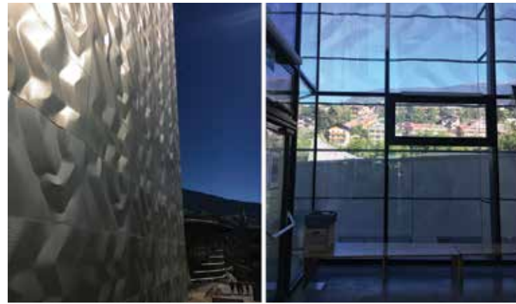
Fig. 2: Kletterhalle Brixen, designed by the architects Wolfgang Meraner and Martin Mutschlechner
