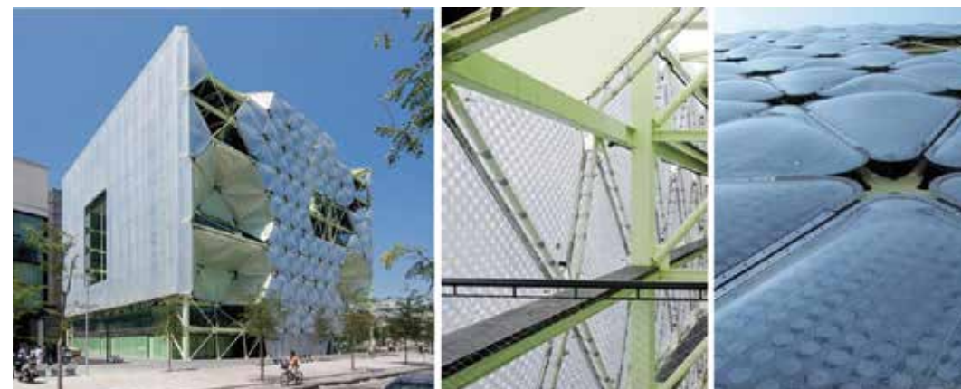
Fig. 3 Example of inflatable adaptive facade (Media ICT building in Barcelona, Spain). (a) General view and (b)-(c) details (figures reproduced from (Marysse, 2016)).
