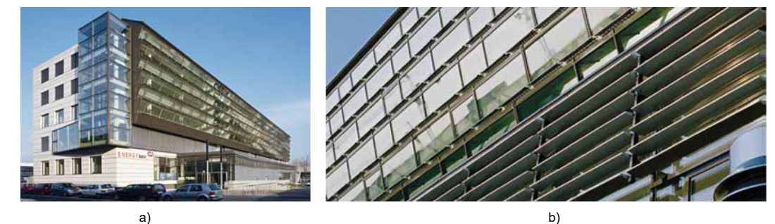
Fig. 6 a) ENERGYbase building (Architekten ZT KG, Vienna, Austria). b) Detail of the South façade.
