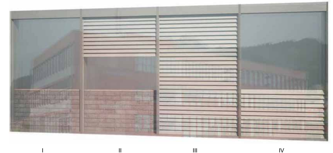
Figure 1 – Solar Energy Balanced Façade with its four main operating states (left to right): I) maximum solar gain, II) glare protection and maximum solar thermal gains, III) maximum sun protection, IV) daylight use and storage protection
