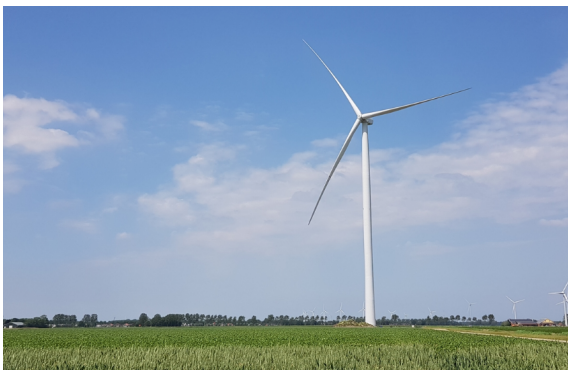
Figure 5.1: TIADE GE 3.8MW research wind turbine [108]
