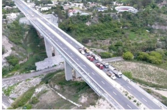
Figure 2. Diagnostic load test in Ecuador prior to bridge opening (Bonifaz et al. 2018).
