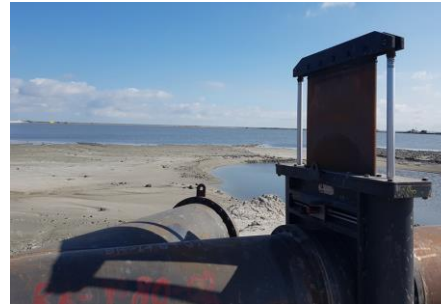
Figure 1-8: A Marker Wadden filling (outlet) pipe, taken on 12-07-2016
