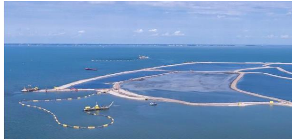
(b) sand berms and initial filling stage
