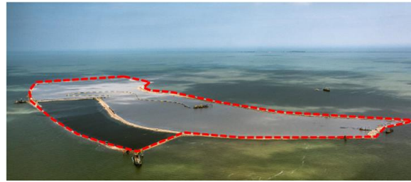
(a) main compartment A construction
