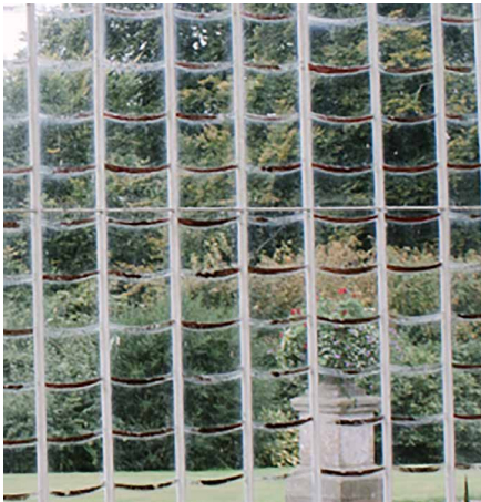
FIG. 4.15 Close-up of 2-side supported overlapping shingles
