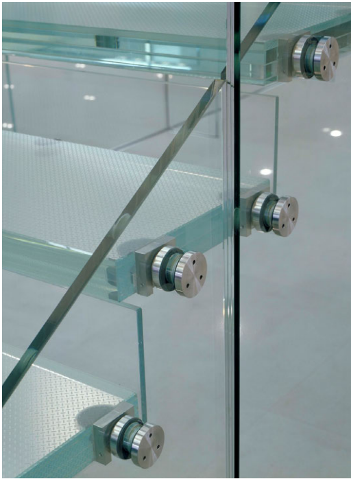
FIG. 7.20 Typically glass structures consist of many layers of glass, connected with opaque fittings that transfer the load.
