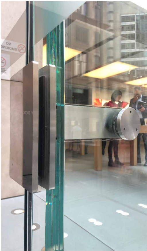
FIG. 3.45 Clamped fitting George street (comparable to CB1)
