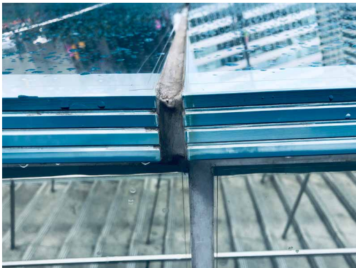
FIG. 3.50 Dilworth Plaza subway entrance, Philadelphia (Kieran Timberlake/EOC)
