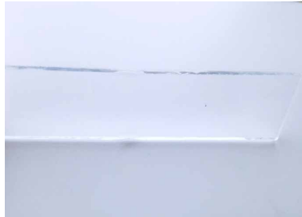
FIG. 6.12 Butt joint manufactured from two sheets of 5mm Borofloat 50mm x 200mm Butt joints are commonly used when connecting glass panels to each other in facade applications. Typically these joints are opaque silicone adhesive joints, which allow to accommodate movement as well. Despite its rigidity, this connection was chosen, as it suggests an opportunity to limit or even mitigate the reflection if light on the edge of the two glass sheets to be connected and hence increasing the perceived transparency.
