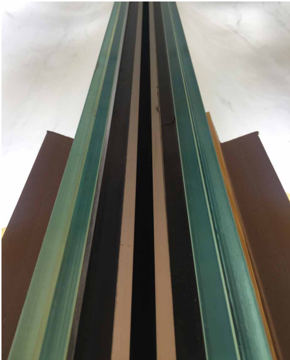
FIG. 3.61 Detail of two half tubes after installation. The glass is protected with an adhesive film
