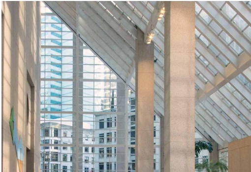
FIG. 7.11 Existing glass clad steel structure 101 California Street, San Francisco, designed by Philip Johnson
