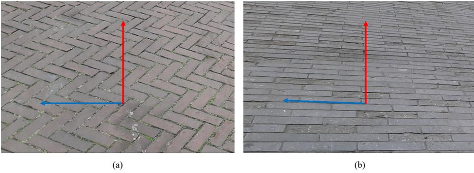
Figure 3.3: The measured anisotropic road surfaces. The red arrow indicates the driving direction ( $\parallel$ ), while the blue arrow indicates the perpendicular direction ( $\perp$ ). (a) Red brick pavement. (b) Grey brick pavement.
