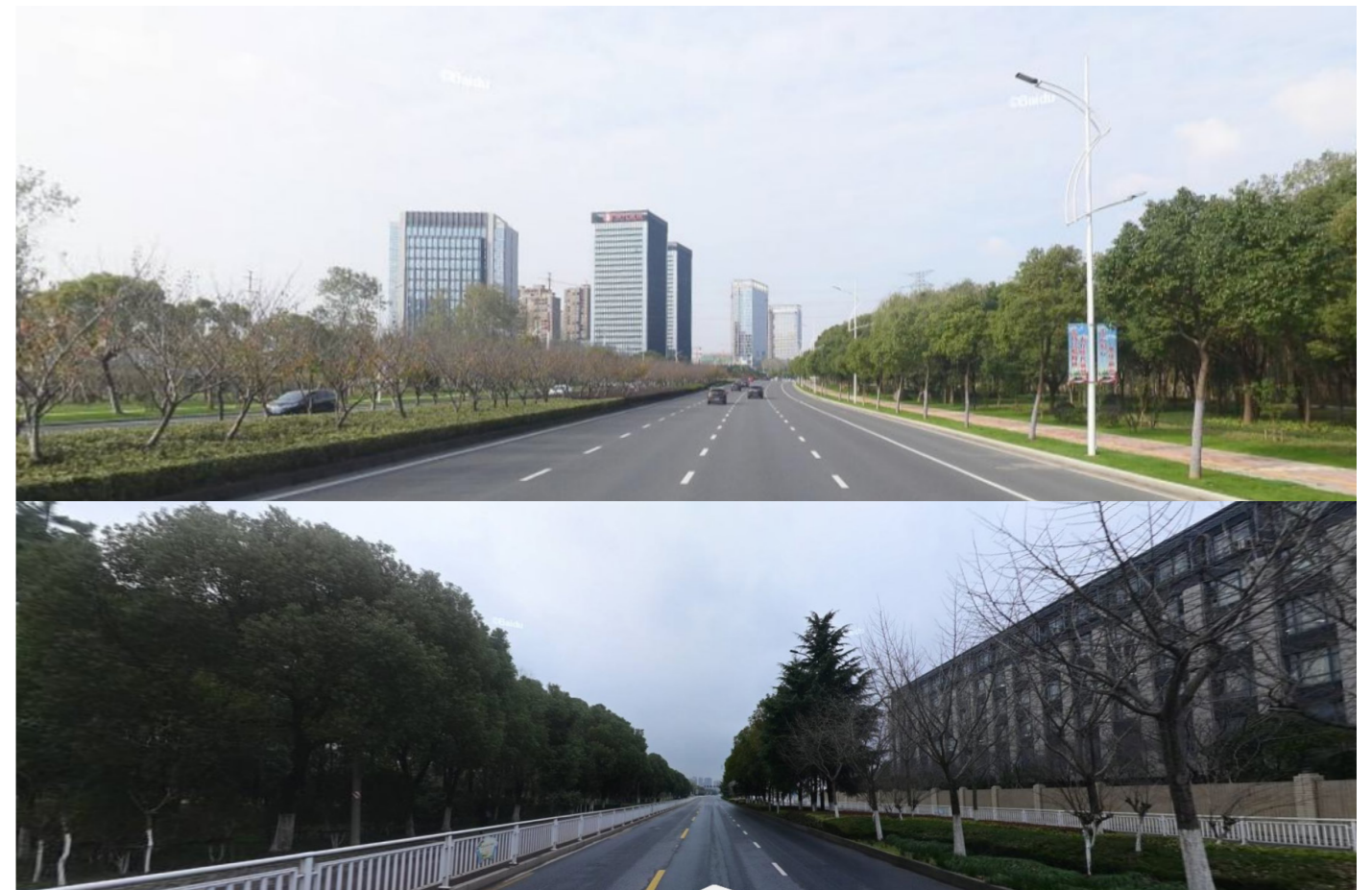
Figure 117. Photo of road condition Source: Baidu Map
