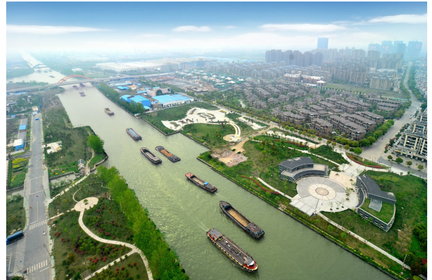
Figure 62. The Grand Canal (San Ta Section)
