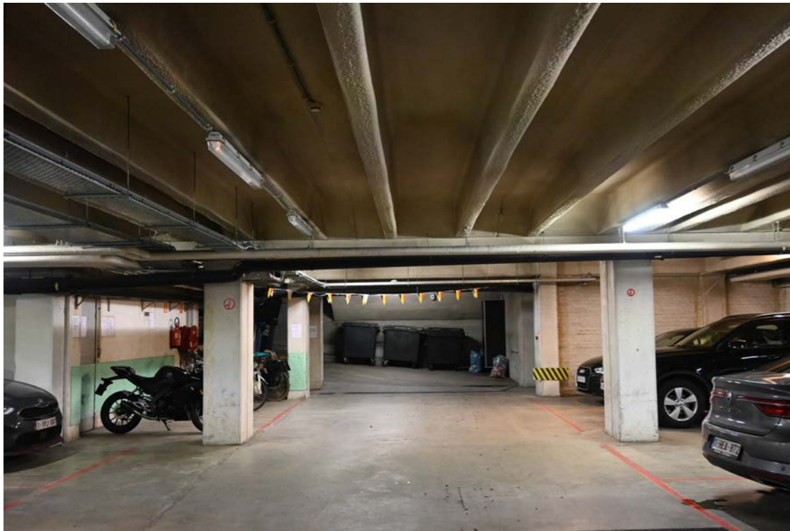
view of the parking space in the basement
