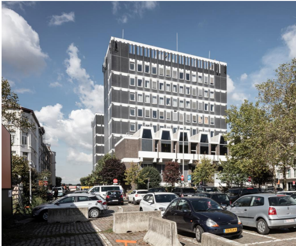
Existing courthouse on site. Credit: Tim van de Velde.
