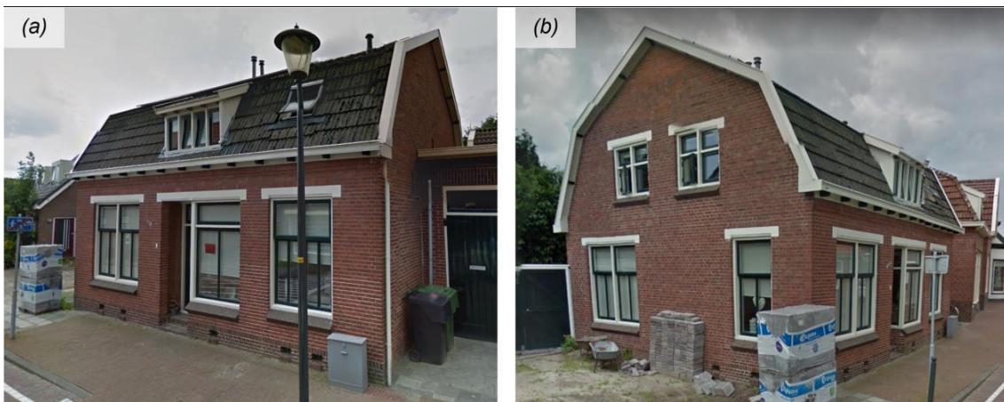
Figure 3: Building views, a) North-East view, b) South-East view (from [3]).
