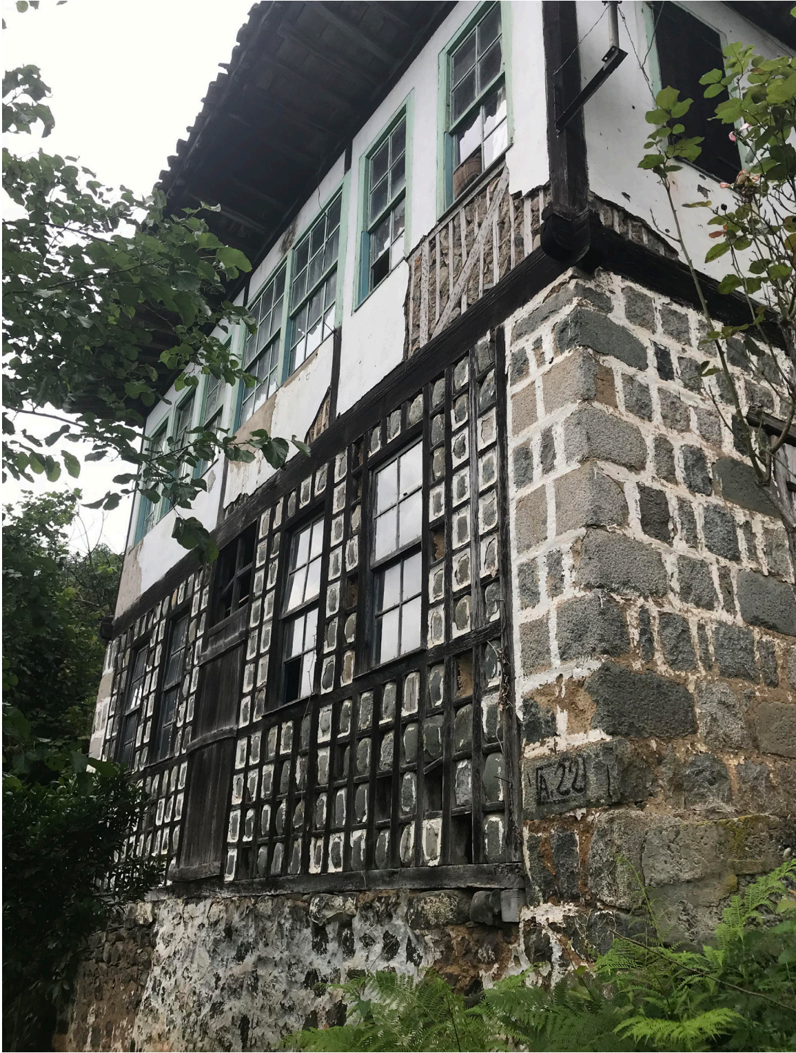
^ Fig. 4 Mixed construction on a building in Hara village (Source: Gül Aktürk, 2019, CC BY 4.0).
