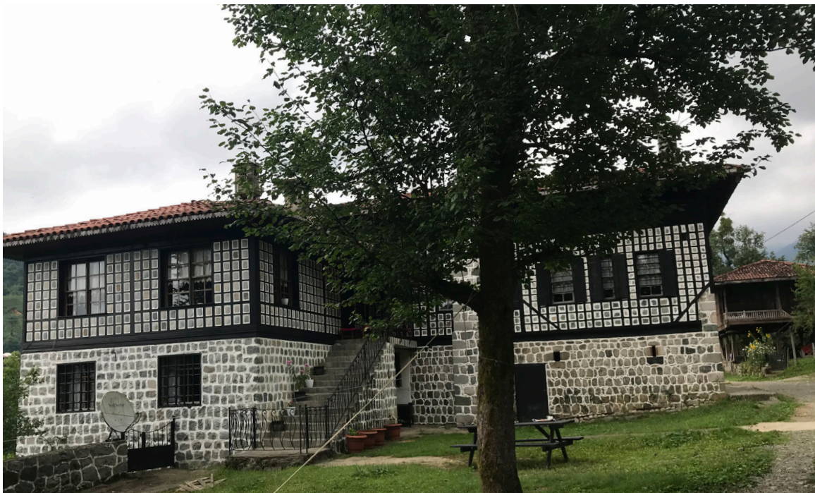
^ Fig. 3 Stone-infilled building in Çağlayan village (Source: Gül Aktürk, Hannah Fluck, CC BY 4.0).
