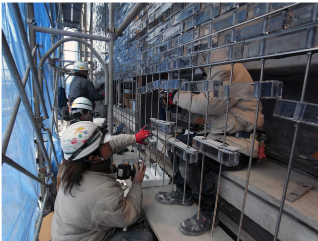
Fig. 20. Assembly of the Optical House . Image credits: Hiroshi Nakamura & NAP.
