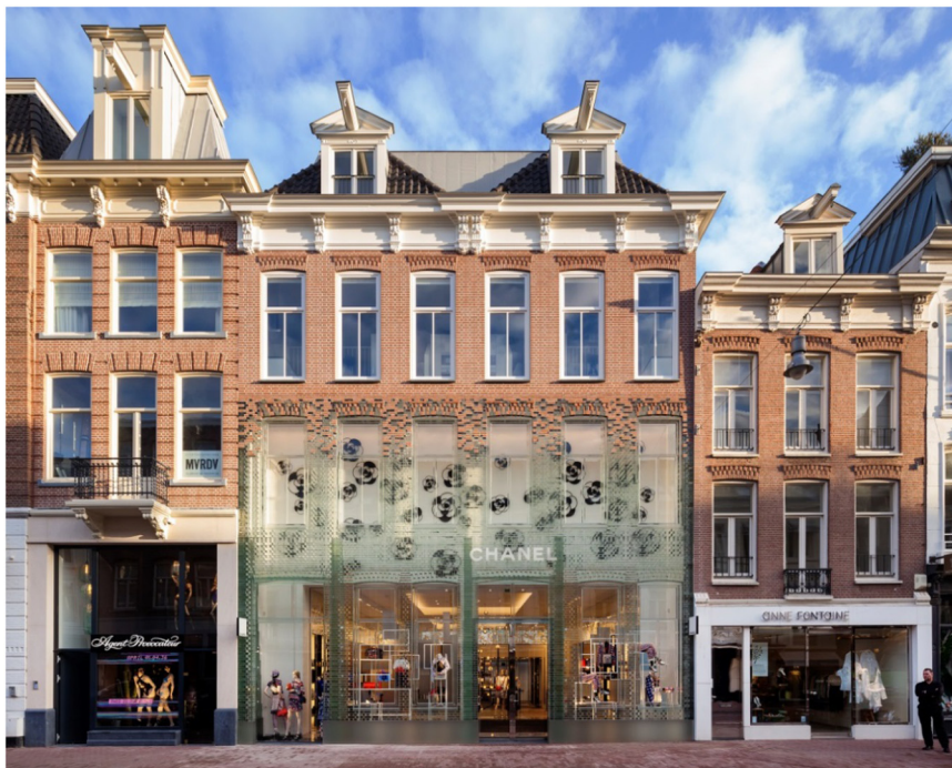
Fig. 2. The Crystal Houses façade by MVRDV Architects, made of adhesively bonded glass blocks. Image credits: Daria Scagliola and Stijn Brakkee.
