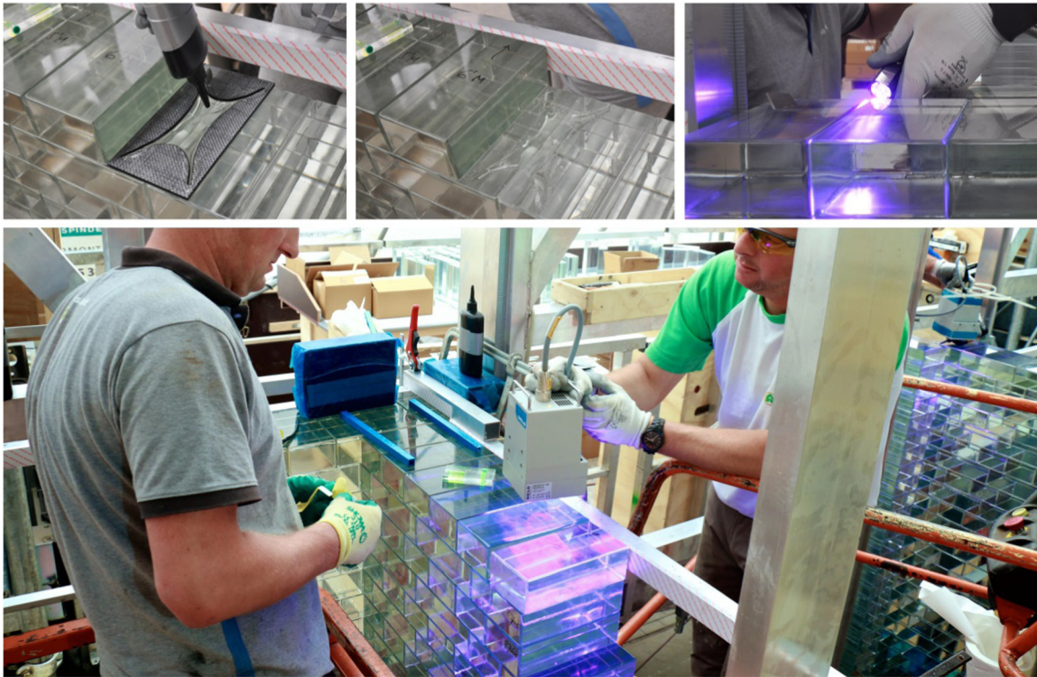
Fig. 32. Bonding and curing of the adhesive at the Crystal Houses .
