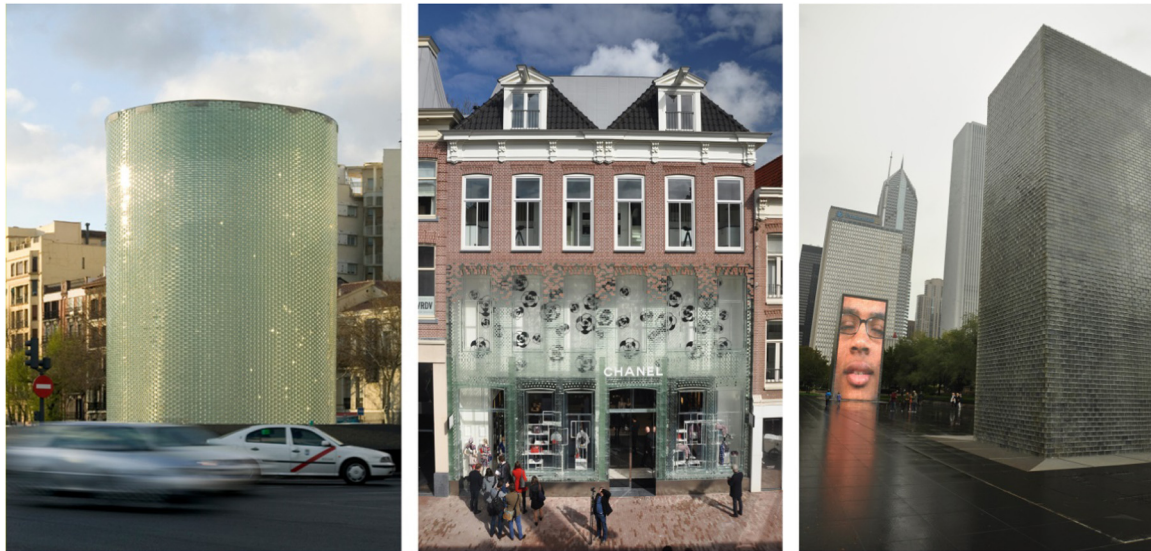
Fig. 16. Characteristic examples of structures employing cast glass blocks: The Atocha Memorial (left) Crystal Houses (centre), and the Crown Fountain (right).
