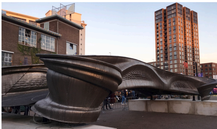
Fig. 1. The MX3D Bridge [9].
