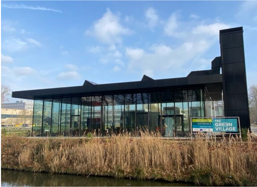
Figure 2-3: Picture of the CONVERGE building with the thermal tower.
