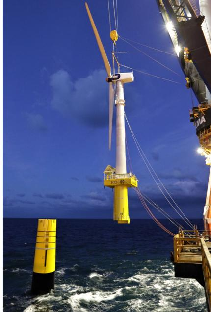
Figure 1.1: Example of a slip joint. [28]
