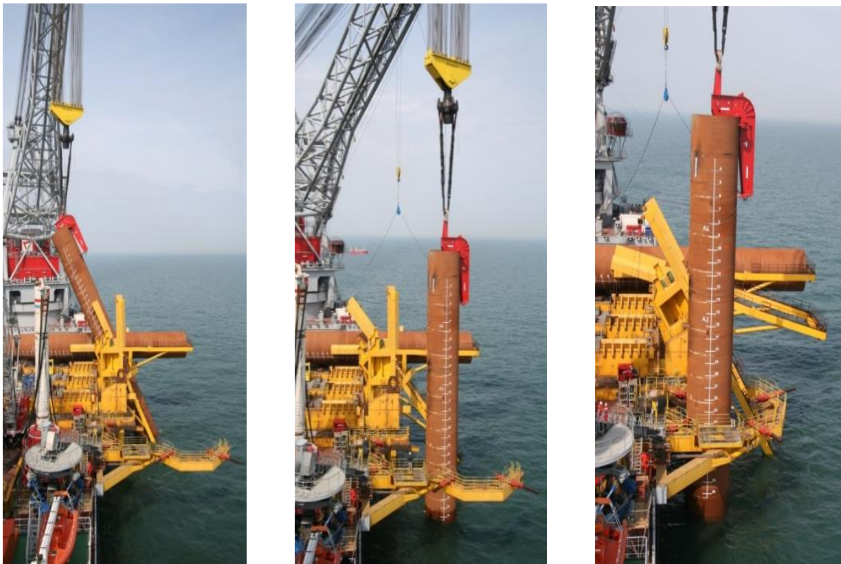
Figure 2-9 - Upending Cradle and the Outrigger [53]
