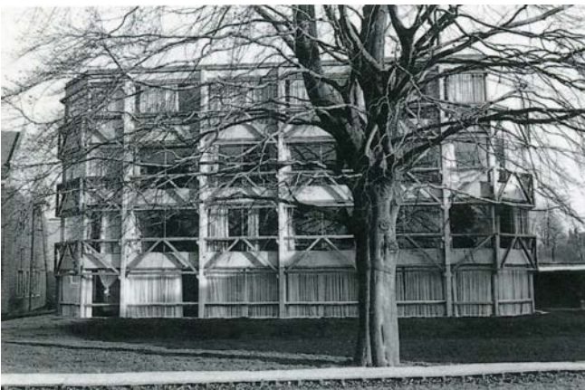
20. Alison and Peter Smith- son, St Hilda's College Dormitory Building, Oxford, 1967-1970, situ- ation
