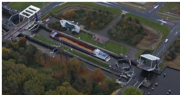
Figure 2 Sea-lock complex Farmsum ("Zeesluis Delfzijl," n.d.)
