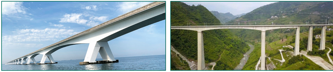
Figure 2.5: Concrete railway bridge examples with varying construction height. Specifically the Zeelandbrug and the Xiangbahe Railway Bridge
