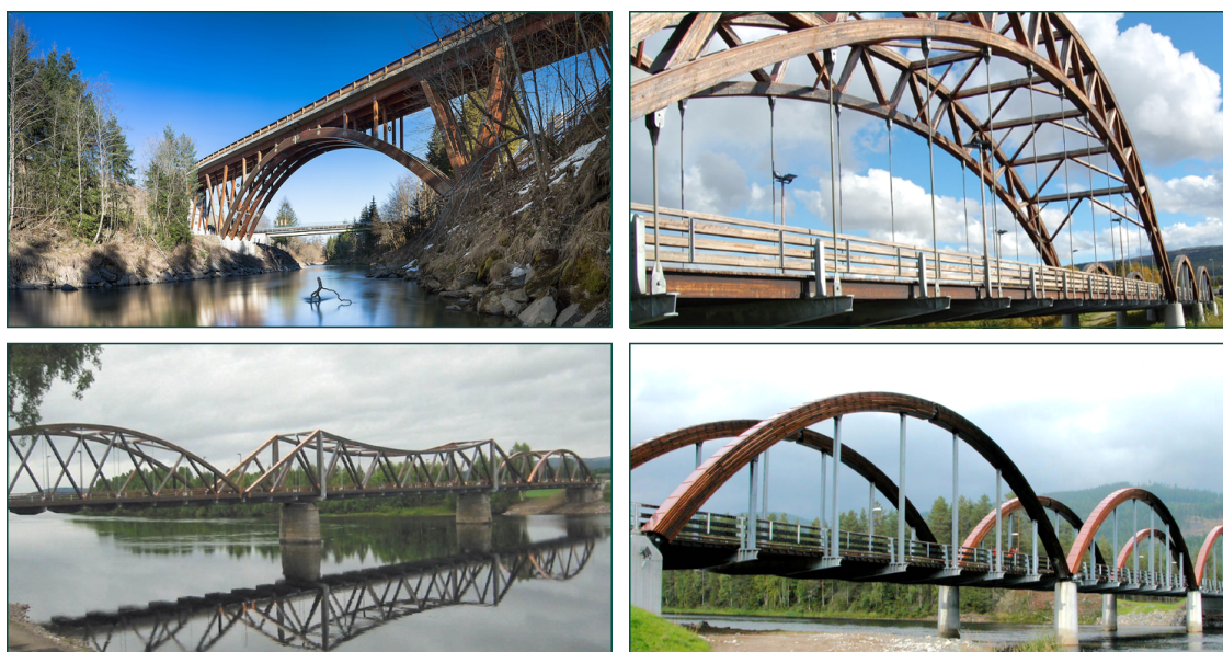
Figure 1.1: Examples of timber bridges. Wennerbrücke has a 45 metre span (top left), Tynnset bridge has a 70 metre span (top right), Flisa bridge also reaches 70 metre (bottom left), and Nyberg Sundbridge spans 40 metre (bottom right) (top left picture is of Pierer (2014), the other three of Aasheim (2019)).
