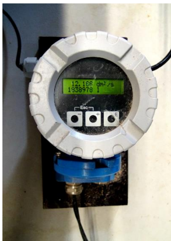
Figure 8; Proline Prosonic Flow 91W discharge measuring tool (Stenfert 2017)
