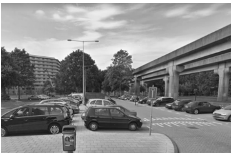
Neighborhood Street (modern neighborhood)
