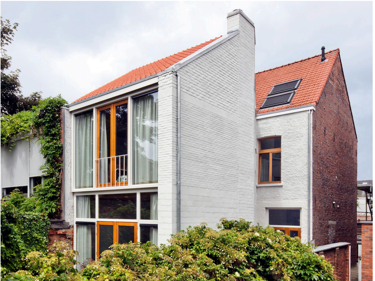
Figure 10, House extension Mortsel seen from the garden (Borghouts, n.d.)
