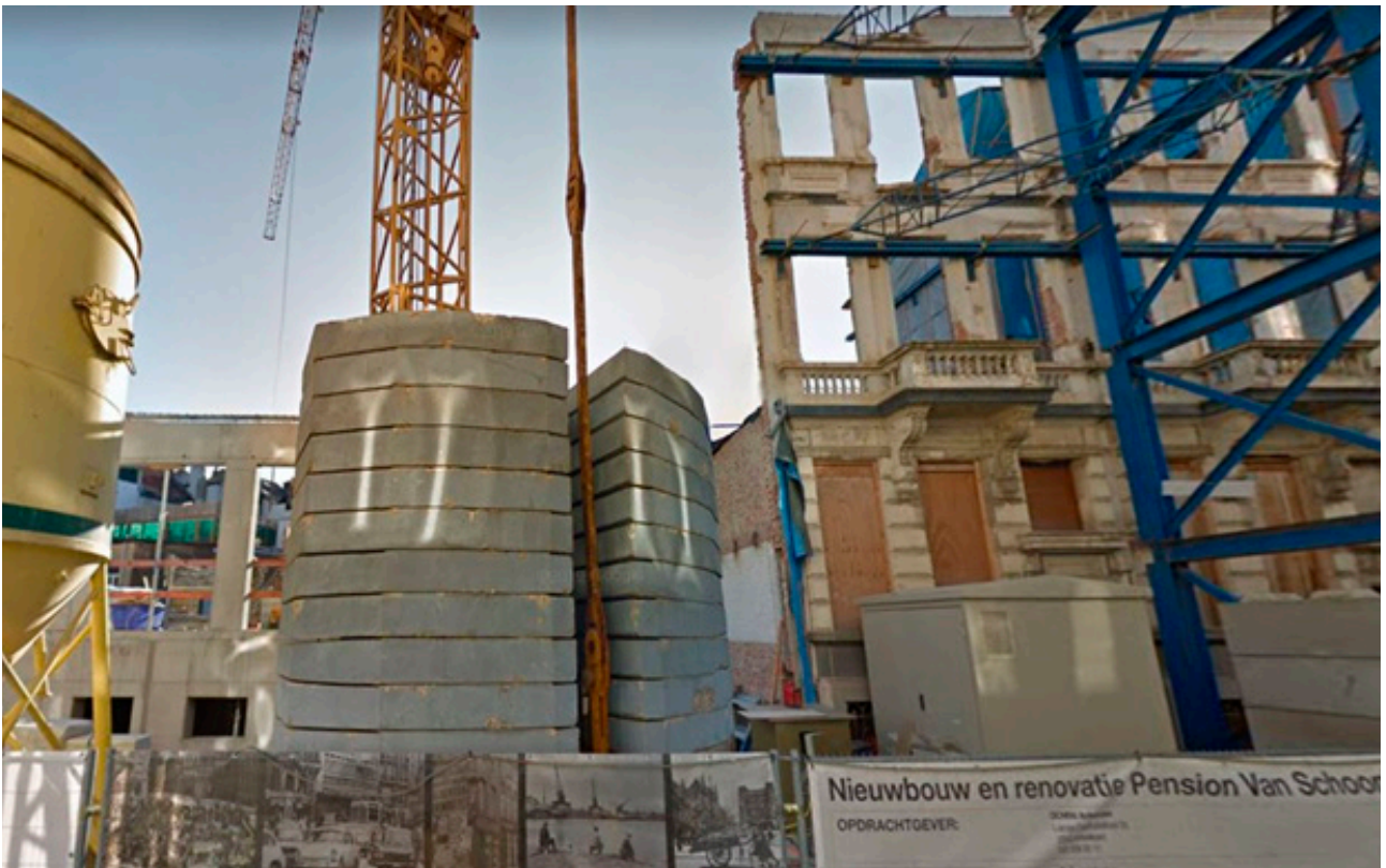
Figure 19, Street View image of Pension van Schoonhoven during construction (Google Maps, 2017)
