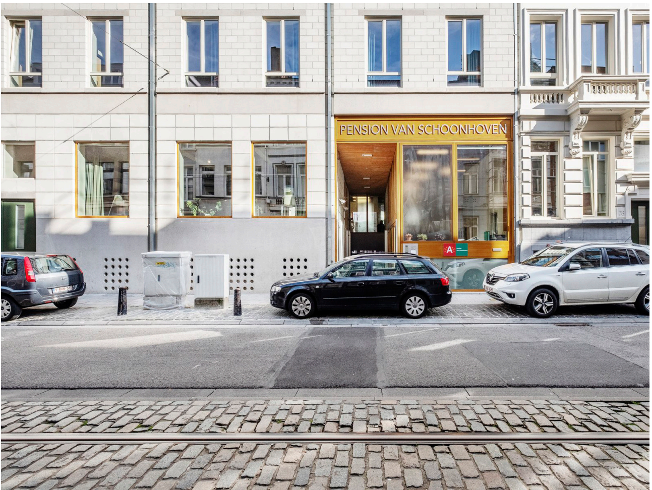
Figure 14, front facade of Pension van Schoonhoven (Claeskens, n.d.)
