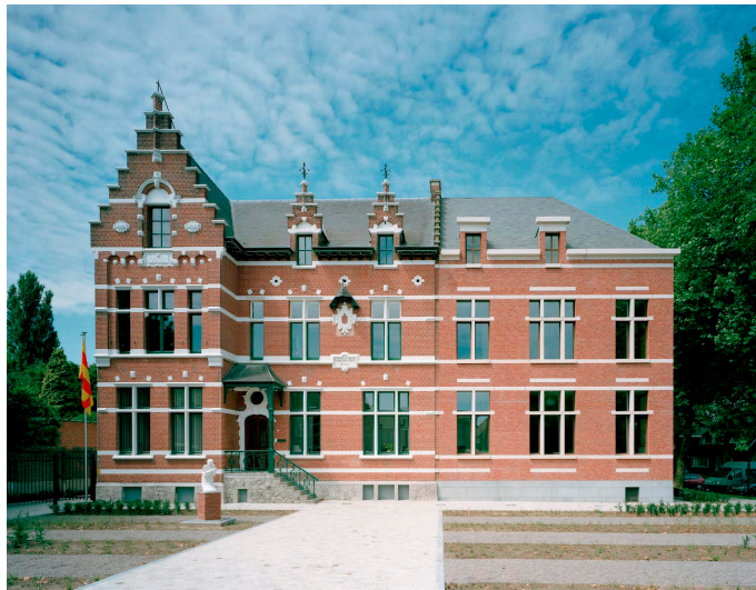
Figure 7, City Hall Niel front facade (Rapp+Rapp, n.d.-c)
