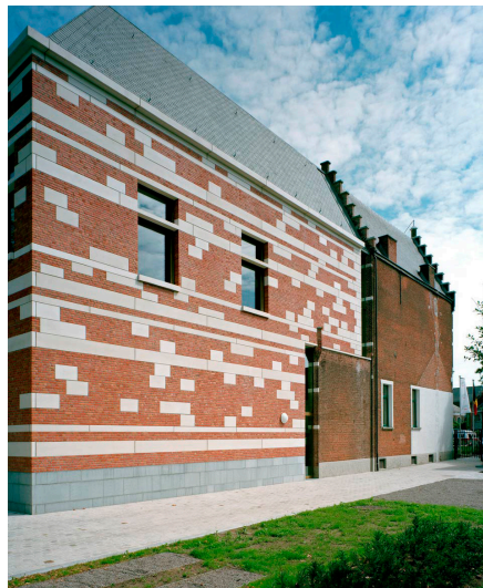
Figure 8, City Hall Niel side facade (Rapp+Rapp, n.d.-d)
