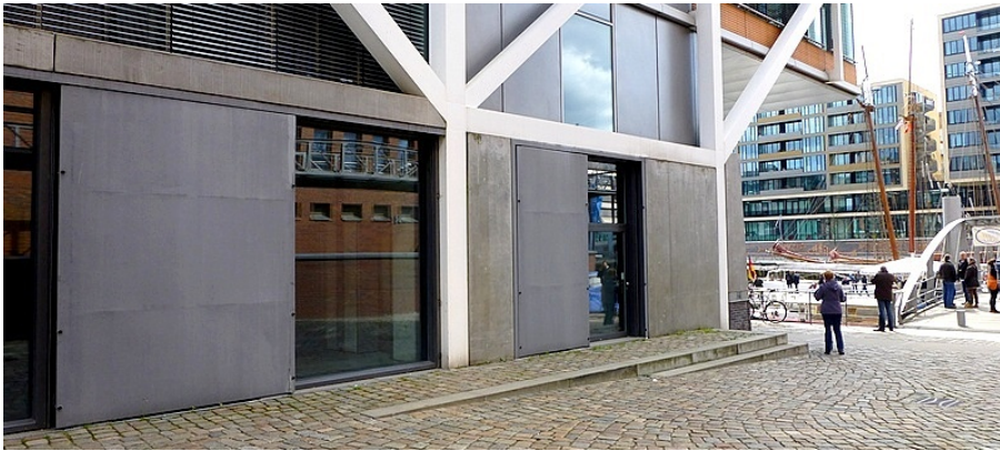
Figure A.20: Hamburg: steel bulkheads can be closed to protect the windows of apartment blocks along the Sandtorkai, May 2012
