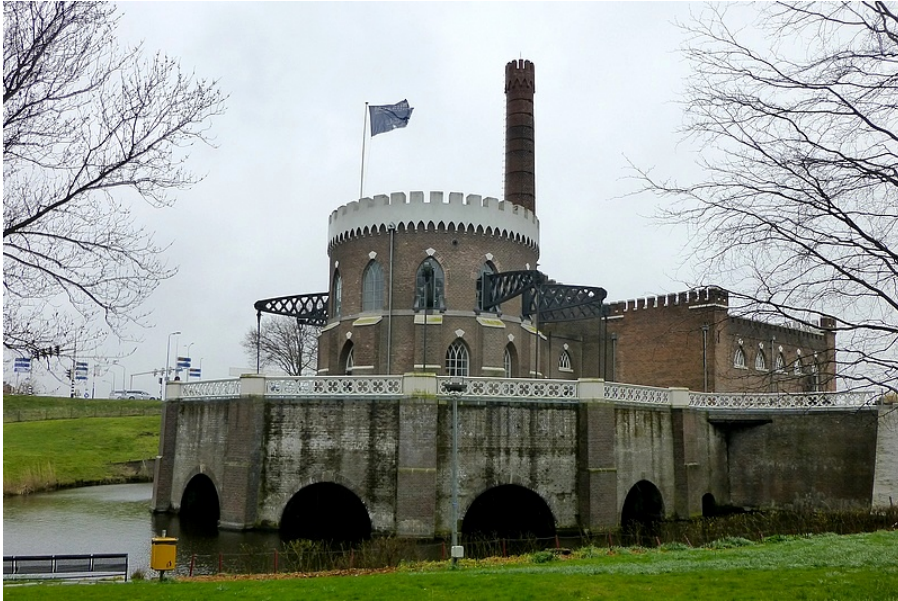
Figure 2.3: Steam pumping station 'The Cruquius', the biggest steam engine on Earth, 2015
