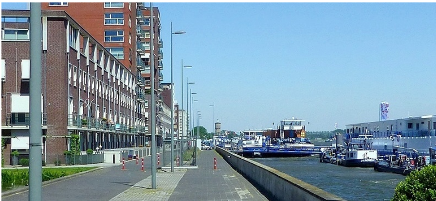
Figure A.10: Zwijndrecht: the Maasboulevard, part of the renewed 'Westkeetshaven', May 2012
