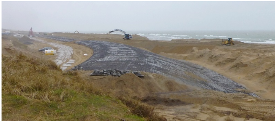
Figure 6.9: Katwijk: construction of the dike-in-dune, February 2014
