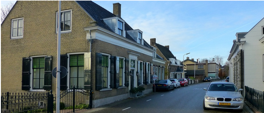
Figure 6.36: Sliedrecht, ribbon development along both sides of the dike, November 2016 (the river is at the left side)
