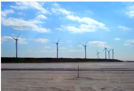
(c) wind turbines on a dike (Maasvlakte, 2011)
