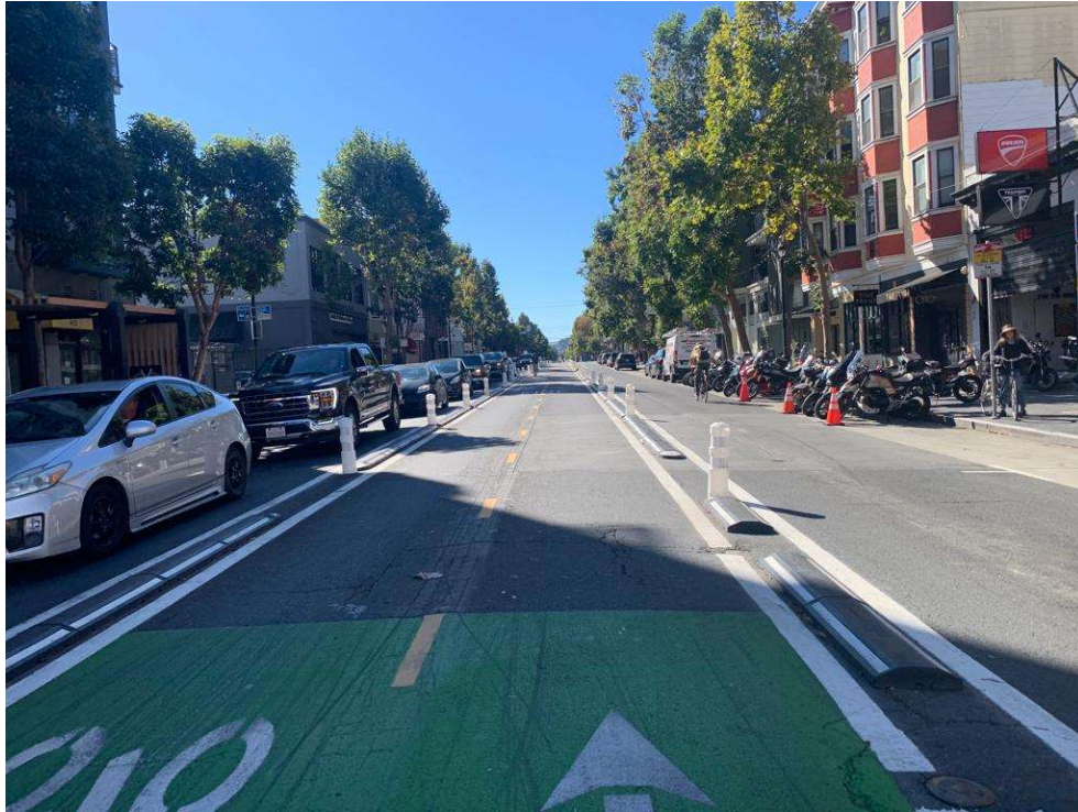
FIGURE 13 - VALENCIA ST BIKE LANE - RUNS DOWN CENTER OF THE STREET
