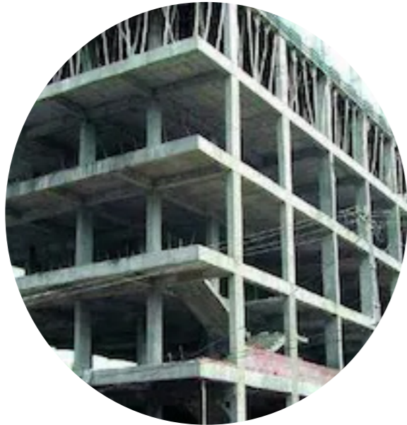
RCC frame structure
