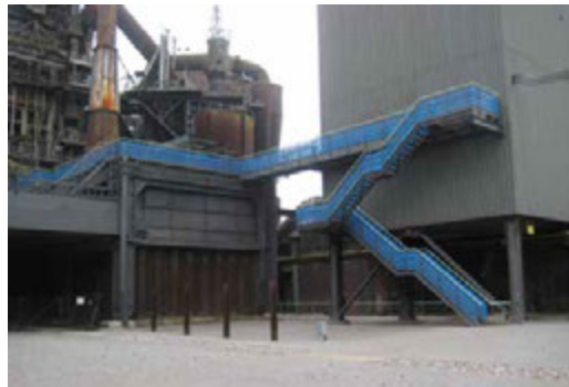
FIGURE 7.22 Blast furnace 5 from Cowperplatz. (Photo: Author).
