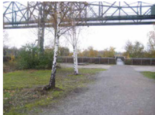
b Bunker roof entrance area. (Photo: Author).
