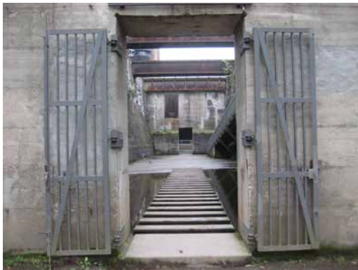
FIGURE 7.31 Bunker passage. (Photo: Author).
