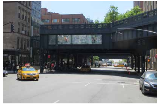
FIGURE 8.33 Sunken Overlook from tenth Avenue. (Photo: Author).
