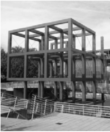
FIGURE 6.44 Folie Escalier. (Photo: Author).
