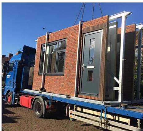
Figure 5.3.9: Façade element Cocoonz renovation method, Source: NBU Nederlandse Bouw Unie, 2016
