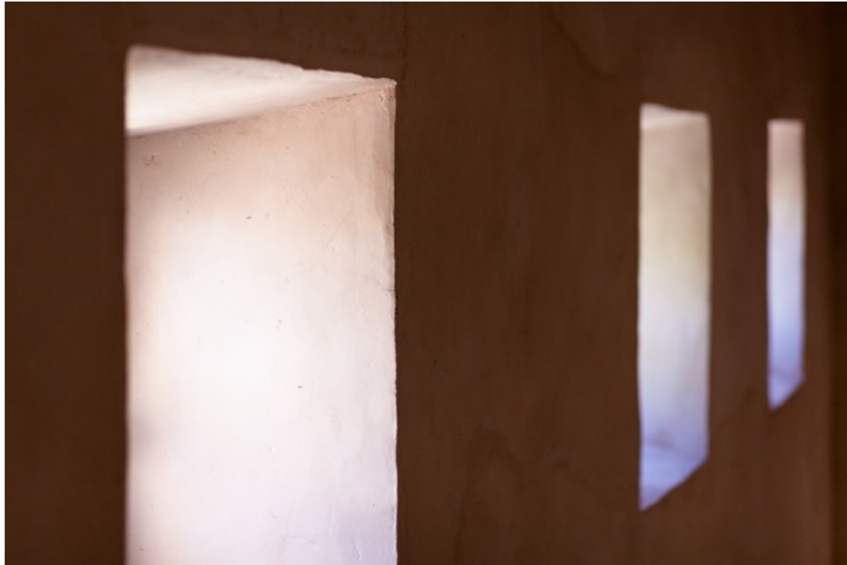
Massive exterior wall - Spain - Passive airco captures night temperatures to keep spaces cool during hot day
