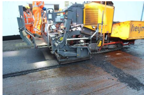
(b) Paving of the new STAC layer
