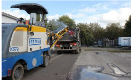
Figure 6.2 Existing pavement removal
