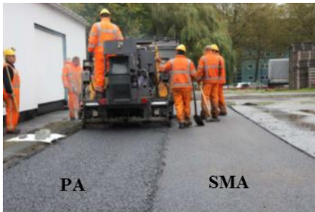
(c) Paving of upper layers (PA and SMA)
