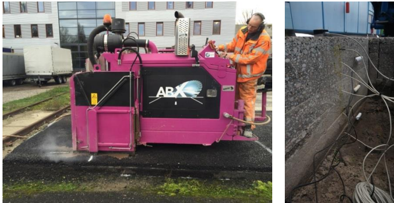
Figure 6.6 Cutting through test section and sensor setup
