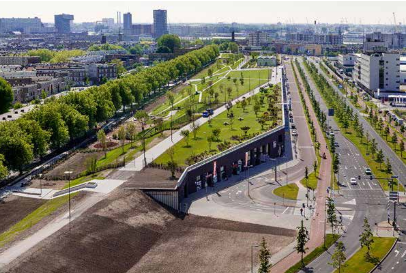
Roofpark Vierhavenstrip, by Buro Sant en Co Rotterdam
