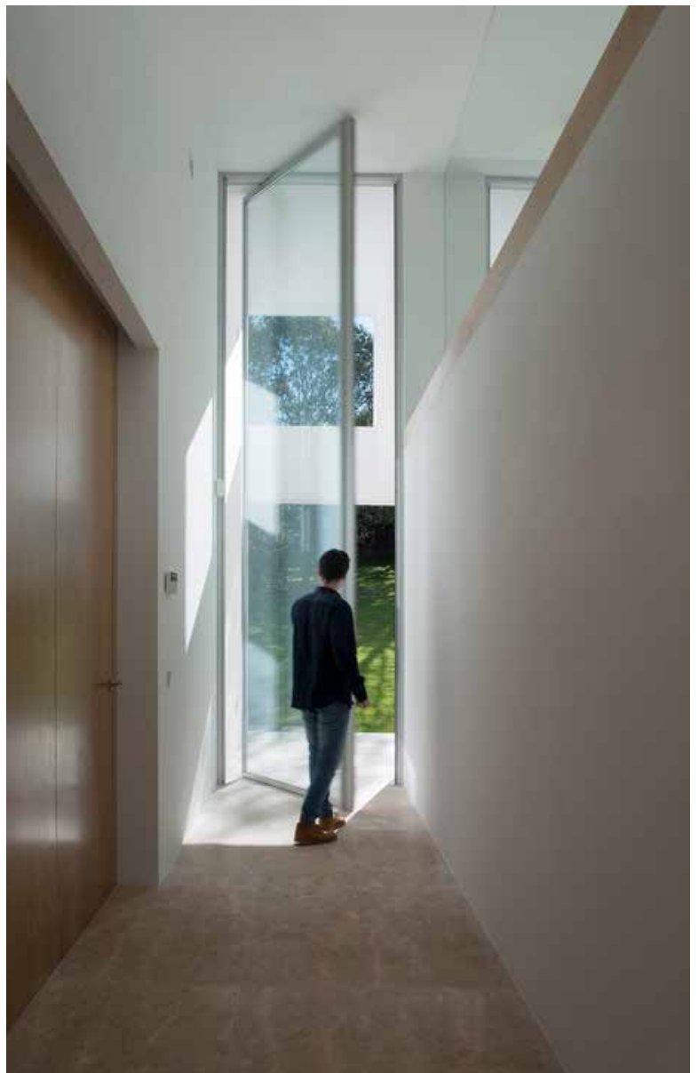
Alternative-3 Pivot hinge window doors
