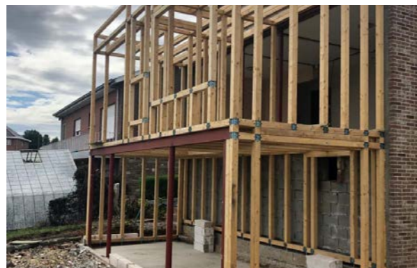
Fig. 12.6 Knoopwerk (n.d.) exterior building
