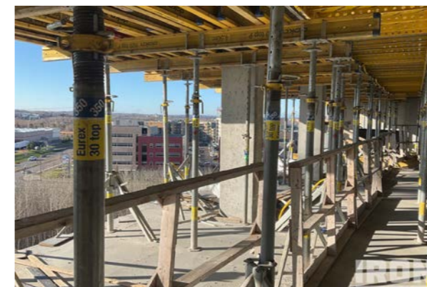
Fig. 10.1 Iron Planet (n.d.) Falsework temporary structure
