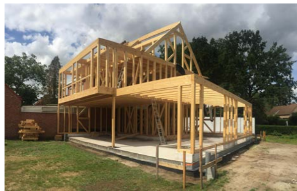
Fig. 12.18 WoodInc (2021) exterior building
