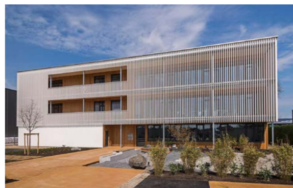
Fig. 12.14 Pollmeier (2023) exterior building
