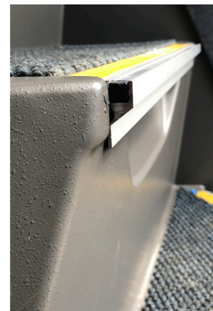
▲ Figure 45 Sharp edges stair steps
