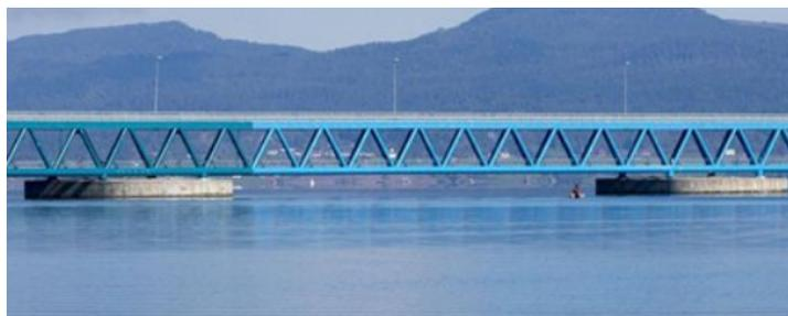
Figure 8.1: Picture of two pontoons of the Bergsøysund bridge.
