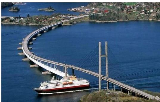
(a) Nord-Hordland bridge, partially fixed and partially floating (Stensvold, B. and Minoretta, A., 2014).
