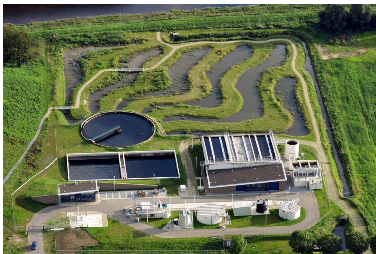
Fig. 1. Photograph of WWTP in Dinxperlo, the Netherlands. The Nereda® reactors are located on the right, attached to the building with the sloped roof. The sludge buffer and the sand filter are located to the right of the Nereda® reactors. The inlet works, including the influent buffer are located at the bottom. The old pre-existing aeration tank and clarifier on the left are now part of a public water garden (on the top).
