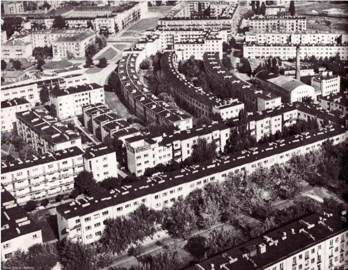
Figure 9. Scan of a picture from a photo album. The picture shows a view to the west of Wilson’s Square in Żoliborz, in the center - the “colonies” (the buildings on the bottom of the scan were designed by Barbara and Stanisław), 1956. Source: Edmund Kupiecki, Warszawa 1960 , page unknown.
