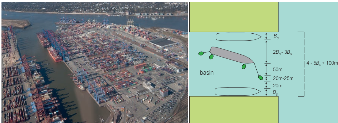
Figure 2.47: Basin width for container terminals (left: Panorama Elbe Hamburg Container In The Air City by www.maxpixel.net is licenced under CC0 1.0; right: image by TU Delft – Ports and Waterways is licenced under CC BY-NC-SA 4.0).
