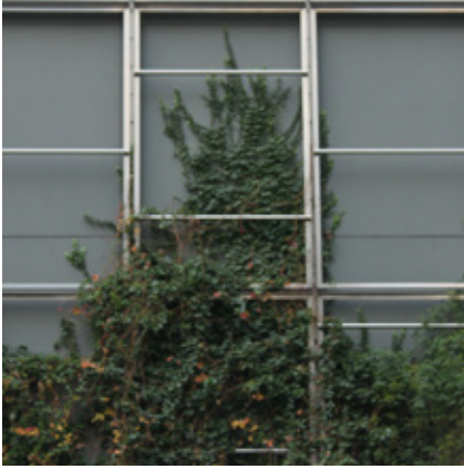
Steel elements and plants Clean and orderly
