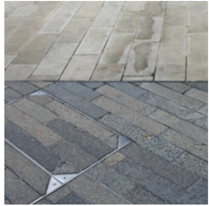
Material transitions No disruptions, clean and orderly
