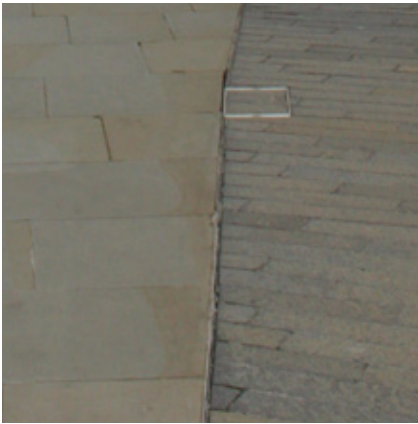
Material transitions Clean and orderly, steel details
