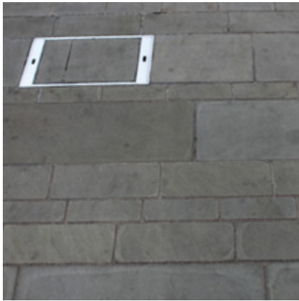
Metal details Clean and orderly, refined details
