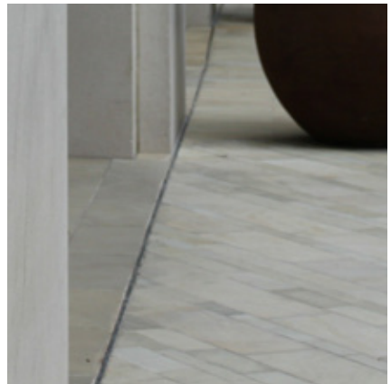
Material transitions Repetition cortensteel and color
