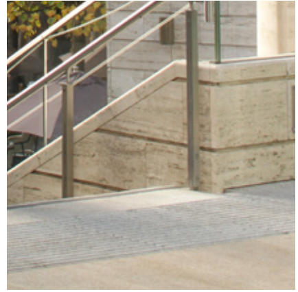
Material transitions Clean and orderly, different textures
