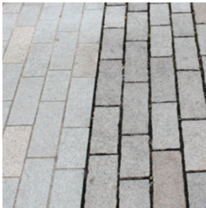
Material transitions Same materials, differences in joints
