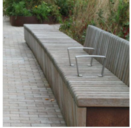
Grey wood, (corten) steel Repetition of materials
