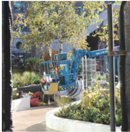
Under construction Disruption
