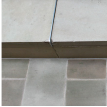
Beige natural stone, metal joints Refined details
