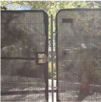
Under construction Disruption
