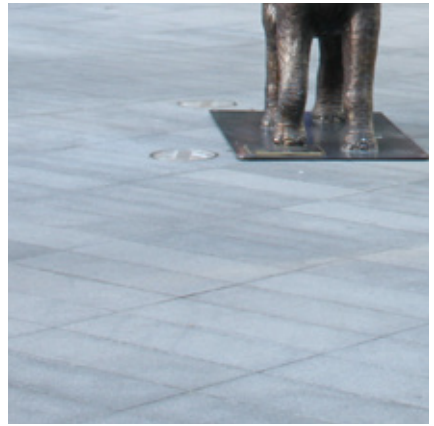
Grey pavement Refined details
