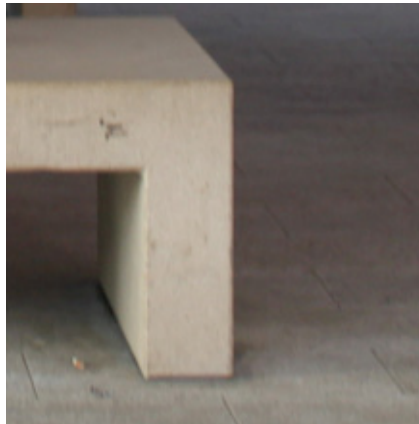
Concrete and grey pavement Repetition of material and color
