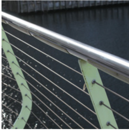
Steel elements Clean details
