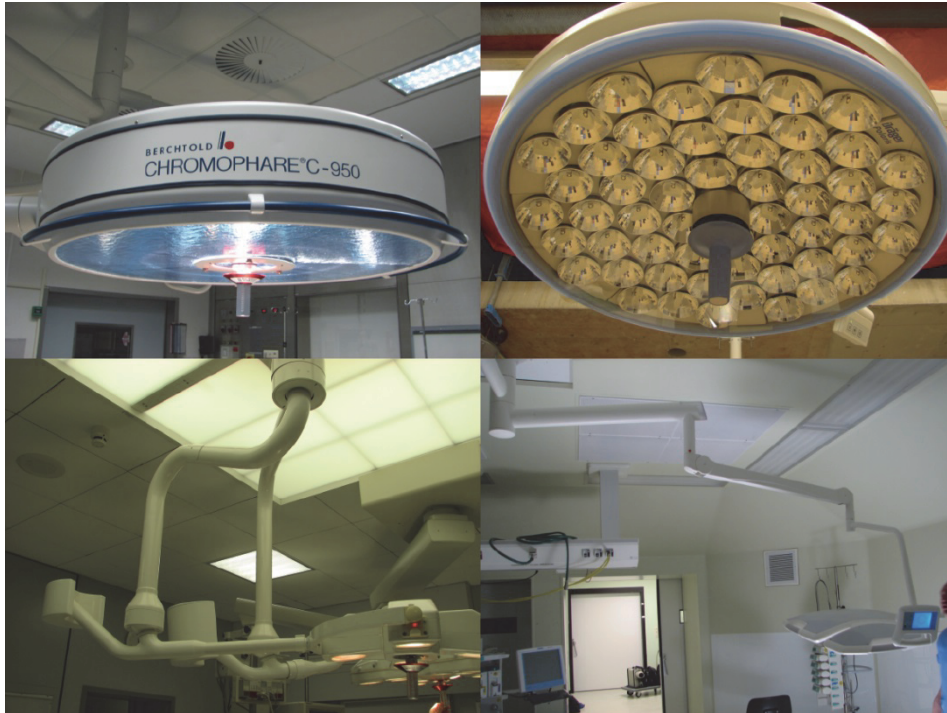
Figure 1.2 a. An older, halogen based surgical light (upper left) and b. a modern LED based surgical light (upper right). C. An older suspension system with a counterweight (lower left) and d. a modern suspension system with a spring-arm (lower right).
