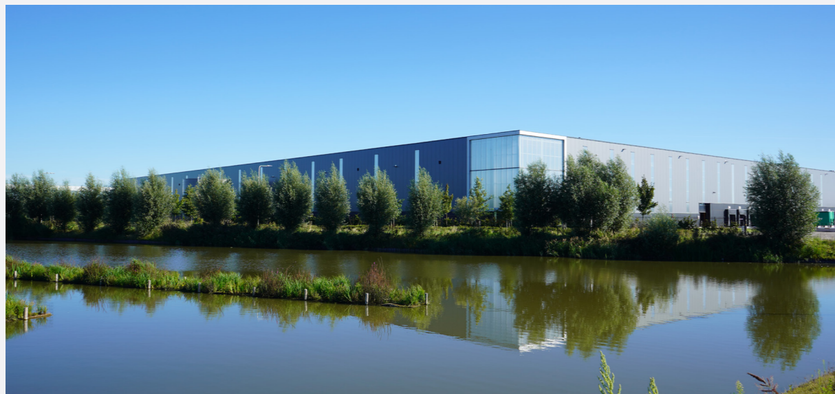
For compensation of the large distribution centres a retention pool is made, to store water that is caught by the large roofs.
