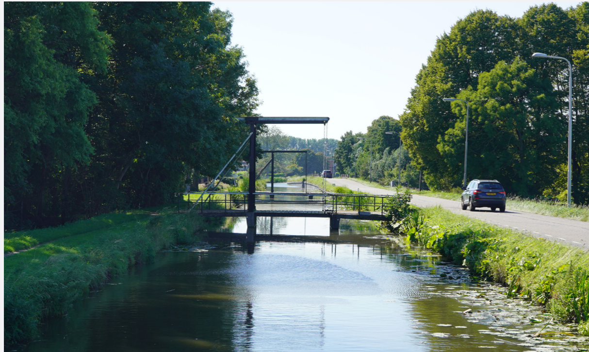
figure 13 - Lift bridges over the Gaag
