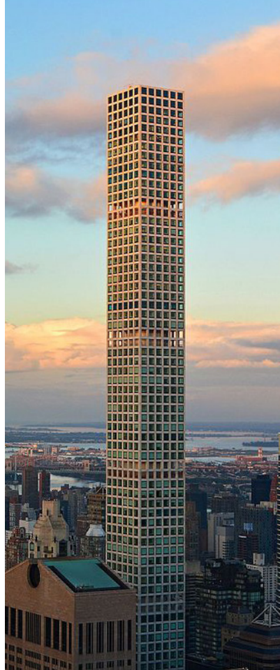
432 Park Avenue - Rafael Vinoly & SLCE Architects
