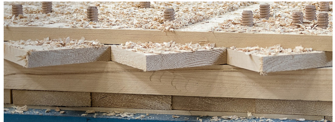
Mechanical lamination with hardwood dowels ( Rombach )
