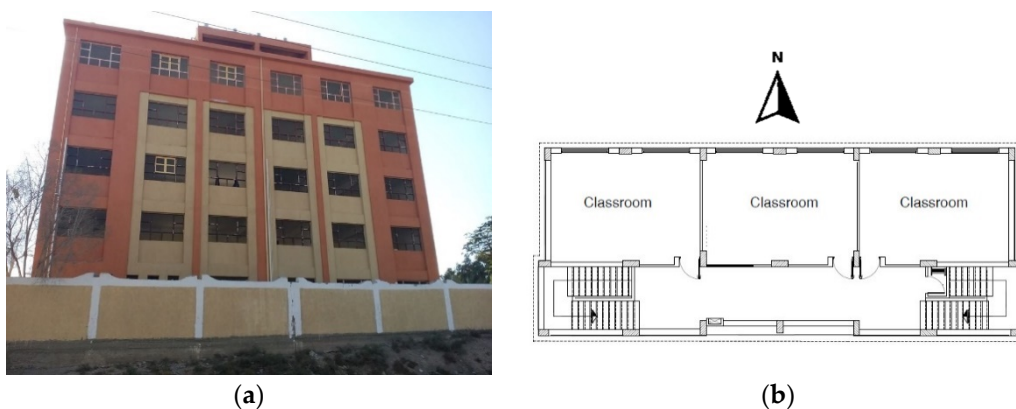
Figure 2. The modeled building. (a) Facade of the school building; (b) Typical floor plan.
