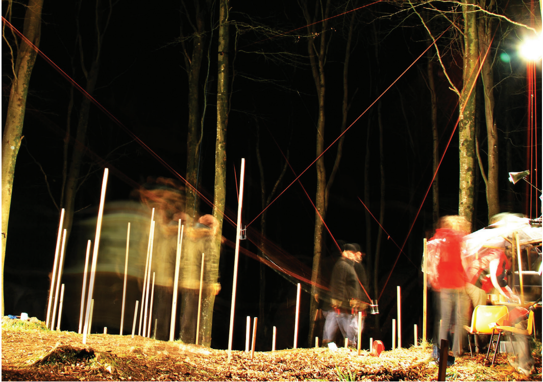
FIGURE 8 Construction and final installation of the field of elements on site, using a web-cam suspended from the trees and a cable robot pointer device.
