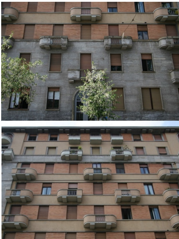
Figure 6 – Details of the lower (at top) and lower part of the Case Study 2's façade.
