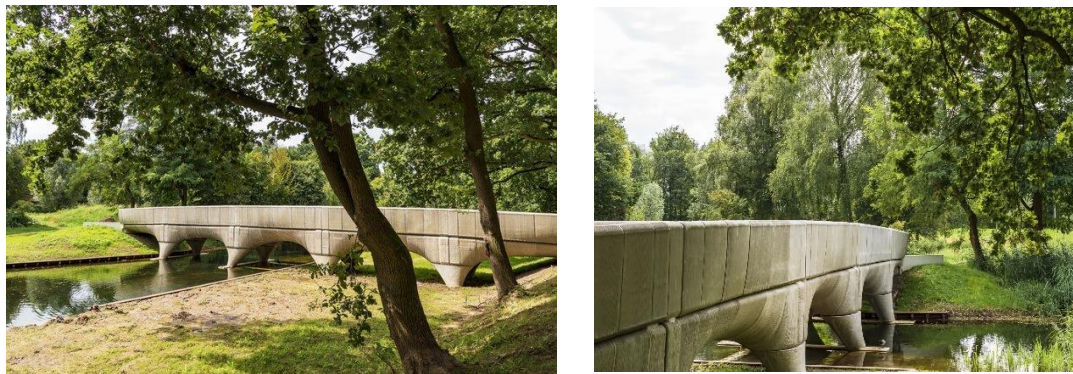
Figure 3: The 3D-printed concrete bicycle bridge in Nijmegen. (Municipality of Nijmegen, 2021)
