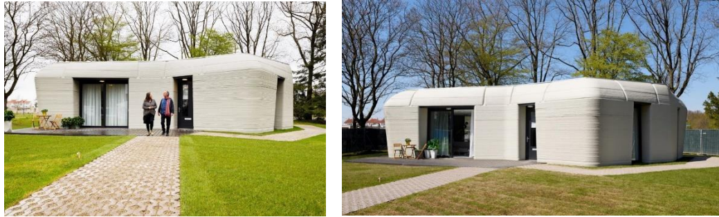
Figure 1: Project Milestone's First 3D Printed House (Ranjit, 2022)
