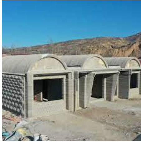
Figure 44: 3 parts of the printed farmhouse (RIC Technology, 2022)
