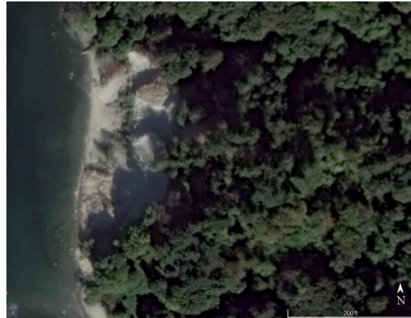
(b) After cliff collapse, on 15 September 2014.
