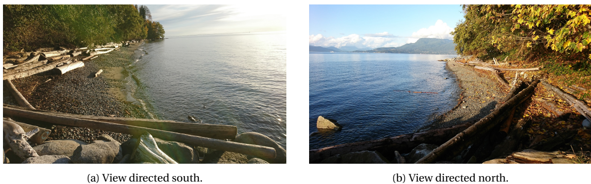
Figure 4.8: Photos at southernmost groyne. Taken on 28/10/2018.
