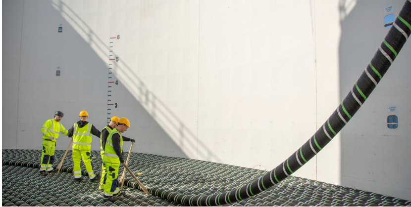
Figure 6.9: Cable loading on a turntable on the NKT Victoria [20]
