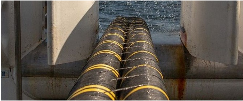
Figure 3.5: Installation of simultaneously bundled DC cables [20]
