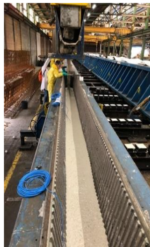
b) Casting of girders
