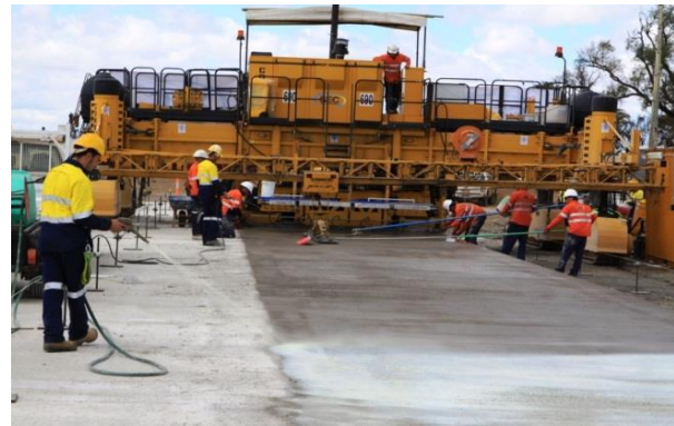
b) BWWA: airport pavement
