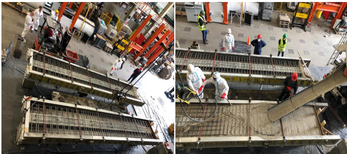
Figure 3.2. Casting operation of the topping over a girder specimen in Ghent University
