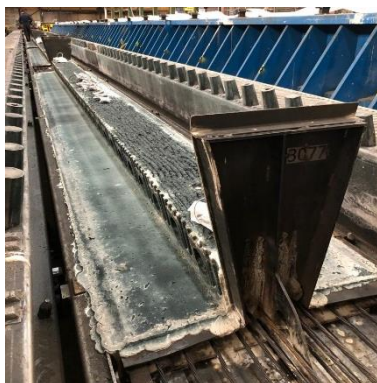
c) Demolding and release of tendons
