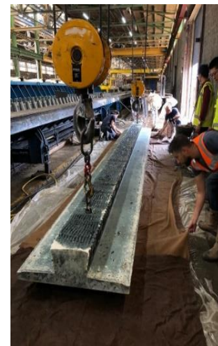
c) Prestressing and demolding
