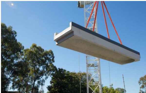
a) Global Change Institute: precast floor elements
