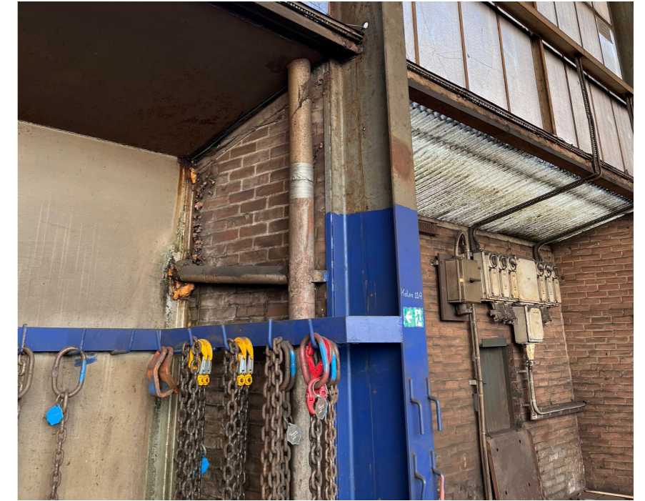
Steel columns (Van Eijck shipyard)
