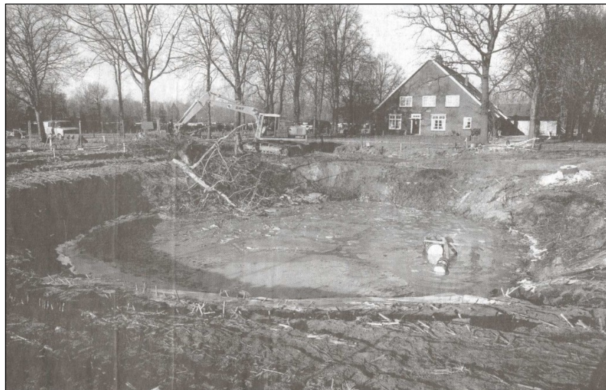
Figure 7.1 Photograph from the sinkhole at the surface above cavern 70 (source: AkzoNobel archive)
